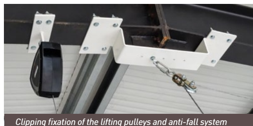
Clipping fixation of the lifting pulleys and anti-fall system
